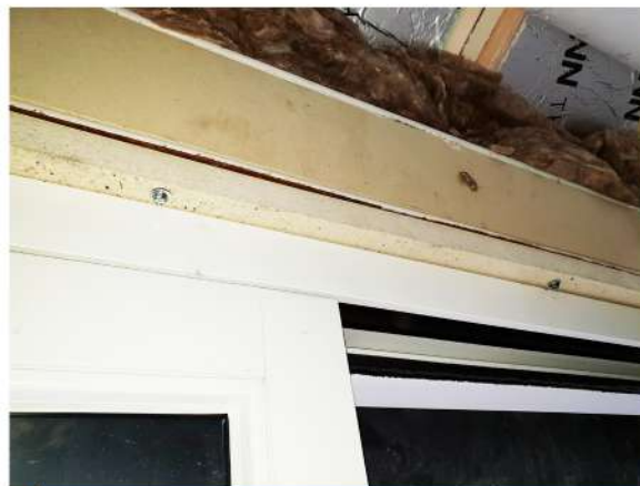
Phonotherm surrounding a steel lintel.
